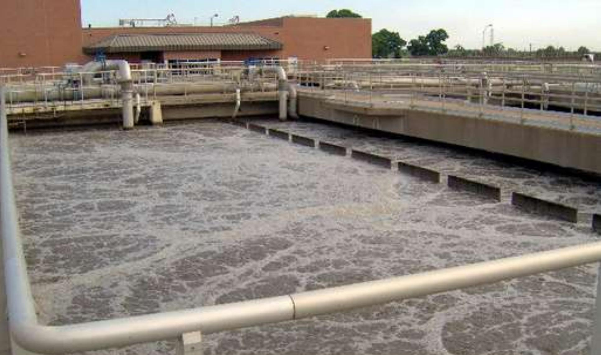
**SECONDARY (AEROBIC) PROCESS = HIGH ENERGY**
