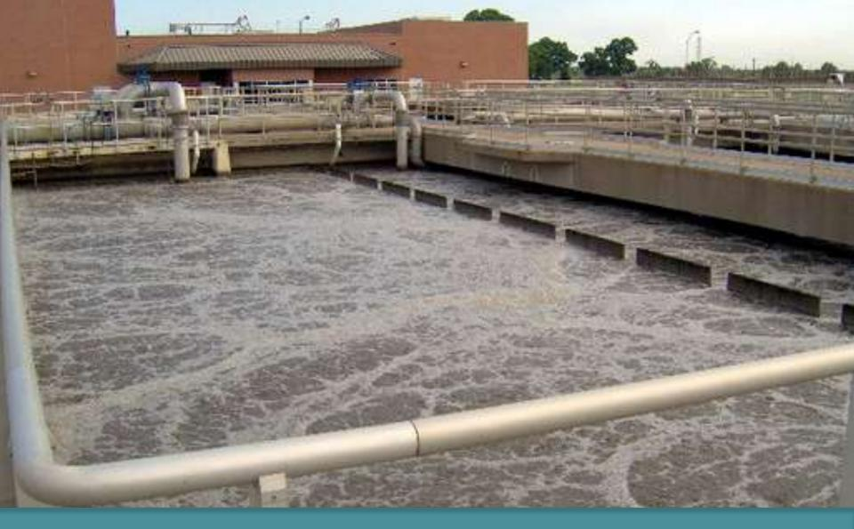
**SECONDARY (AEROBIC) PROCESS = HIGH ENERGY**
